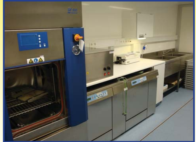
The equipment in the sterilization is of high quality and high capacity.
